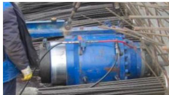
4-rasm: “Post tension” – keyingi zo‘riqtirish
