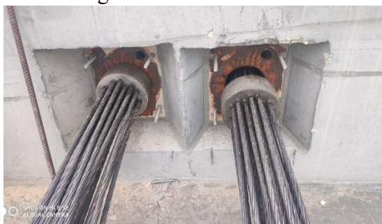
4-rasm: “Post tension” – keyingi zo‘riqtirish
